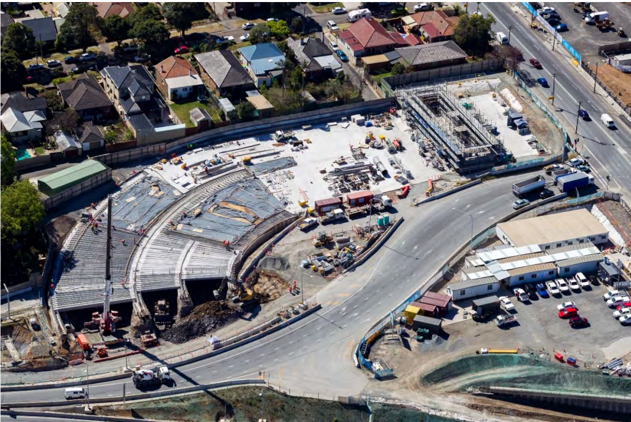
Figure 6-7 New M4 tunnel cut and cover structures
