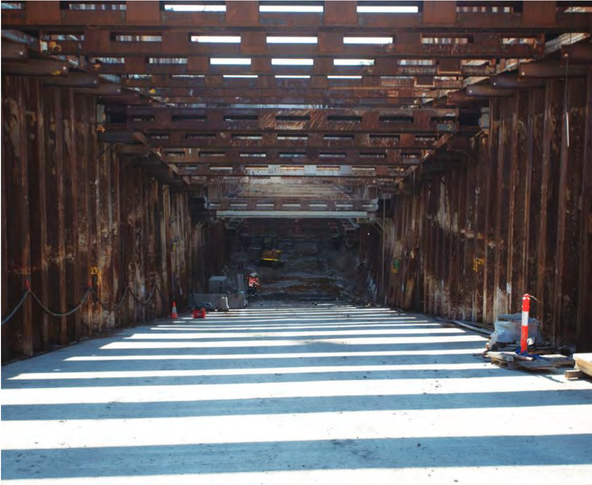
Figure 6-2 Example tunnel access decline
