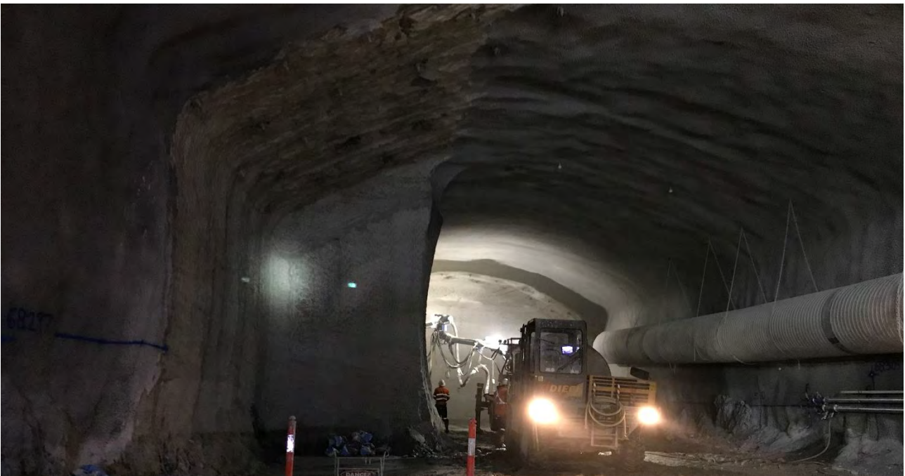
Figure 6-5 Example of tunnel shotcreting
