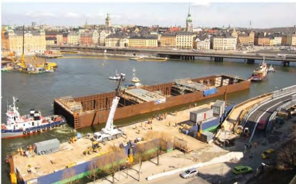
Floating steel shell unit arriving at casting facility for concrete construction. *
