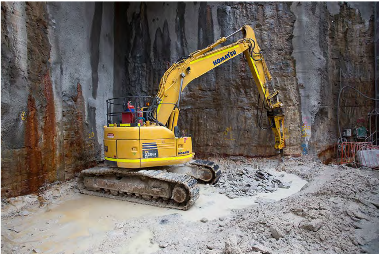
Figure 6-6 Example of rock hammering
