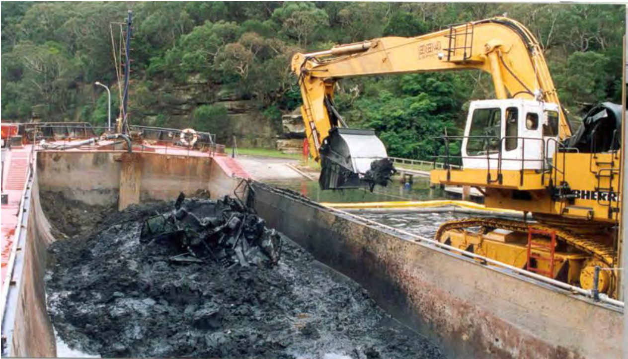
Figure 6-14 Example of an excavator fitted with a closed environmental clamshell loading into a hopper barge (Source: supplied by Royal Haskoning DHV, 2020)
