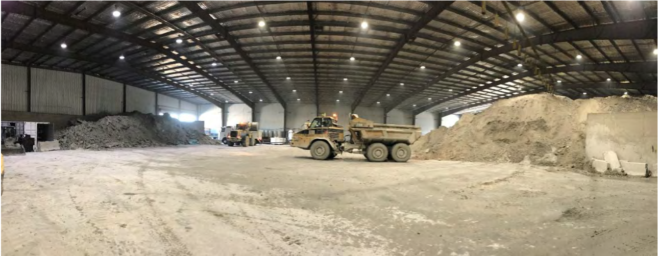
Figure 6-3 Example from within an acoustic shed constructed for the New M4 tunnels
