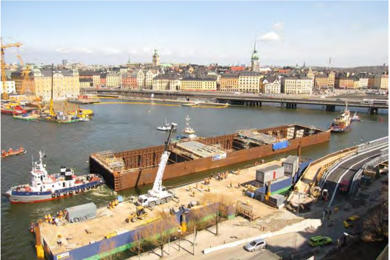
Figure 6-16 Example of a casting facility for the Soderstrom Tunnel, Stockholm (Source: TunnelTalk, 2013)
