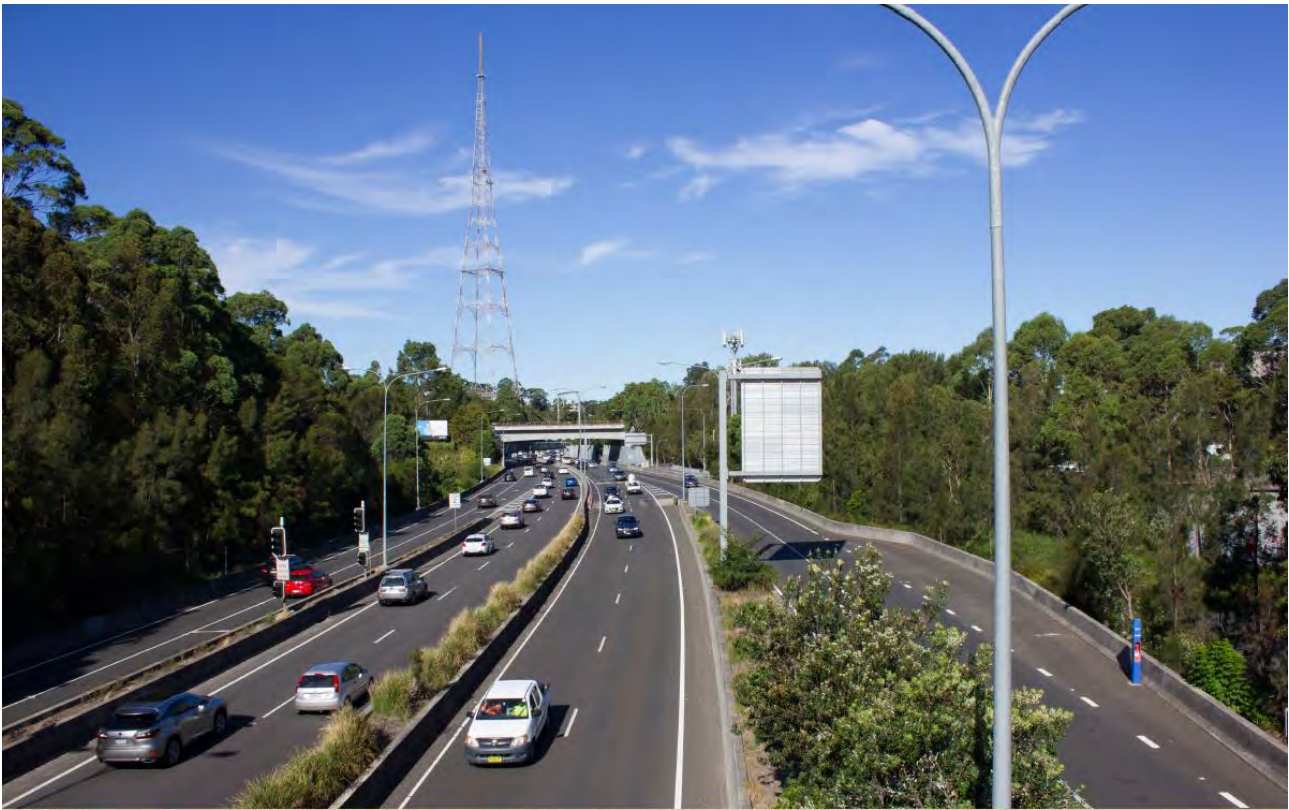
Figure 22-17 Existing view east over Gore Hill Freeway from Hampden Bridge towards the motorway facilities and ventilation outlet
