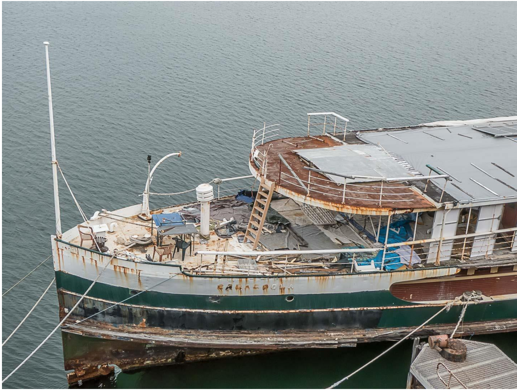
Fig. 13 Baragoola on 4/9/2021 The clutter of work that has been in progress for thirteen years
