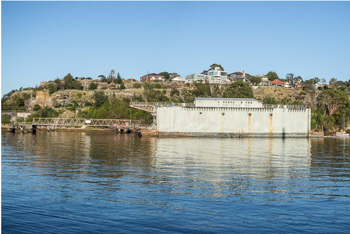
Fig.17 Noakes Floating Dry Dock on 29/12/2014
