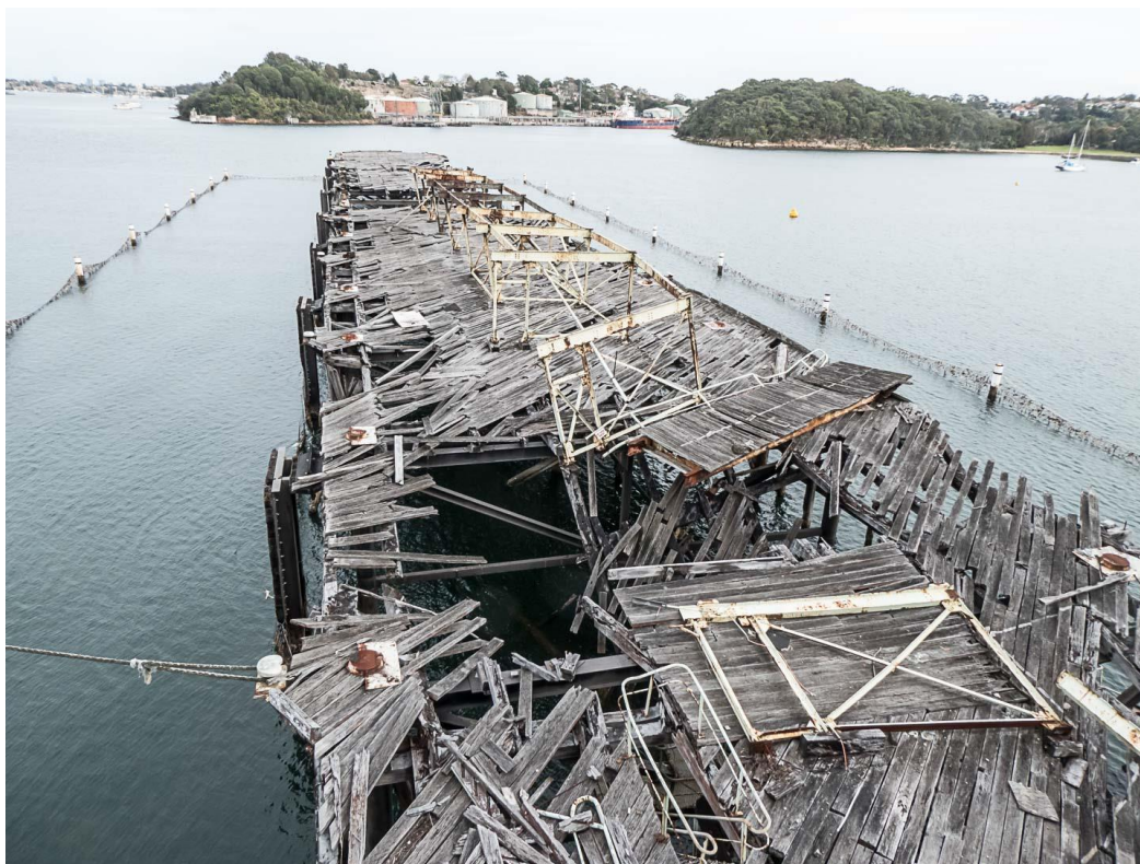
Fig. 15 The remains of the Coal Loader wharf on 4/9/2021
